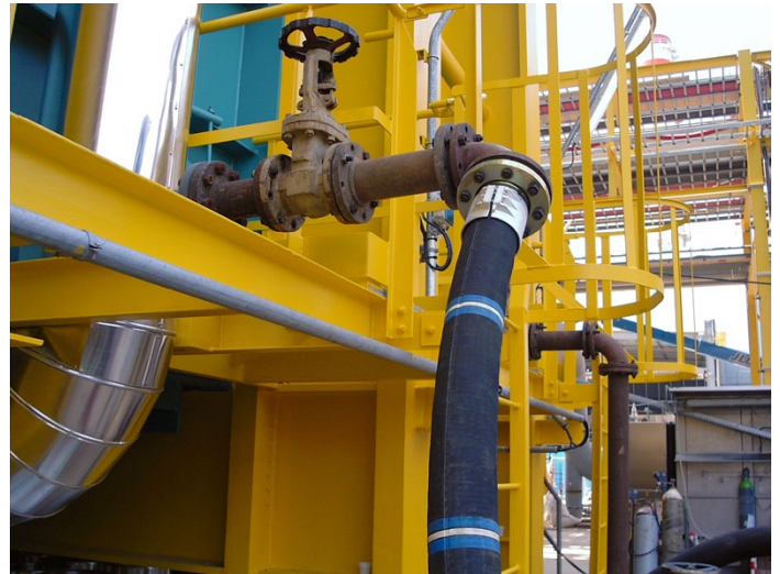
UTS flanged hose / permanent high pressure + high temperature use, alkaline solution - Italcem, Italy
