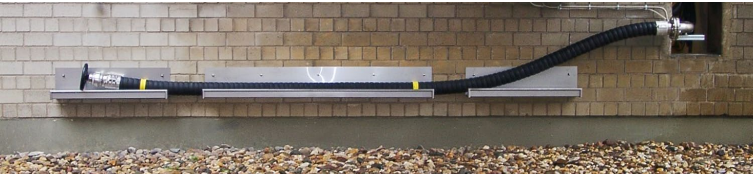
DDC couplings / special application / environmentally friendly mobile 'latent heat storage system' with hot water - LaTherm, Germany
