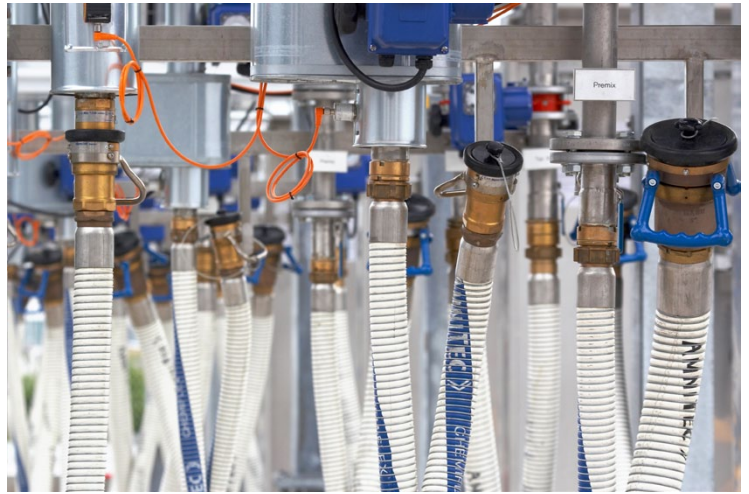
DDC couplings and FWS composite hoses / airport de-icing facility - Goehler, Germany
