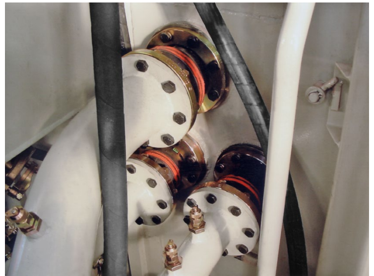
ERV ROTEX / cool water line seagoing ship - Zacharias Anlagentechnik, Germany
