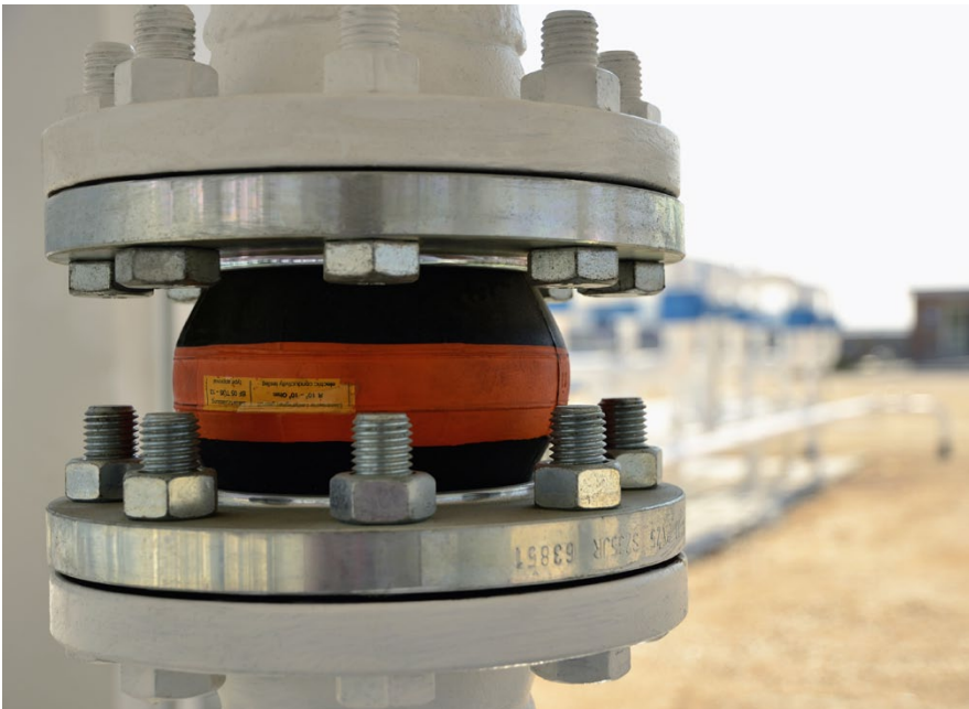
ERV-OR 100.25 Orange Band expansion joint / storage facility Porto Romano - Primagas, Albania
