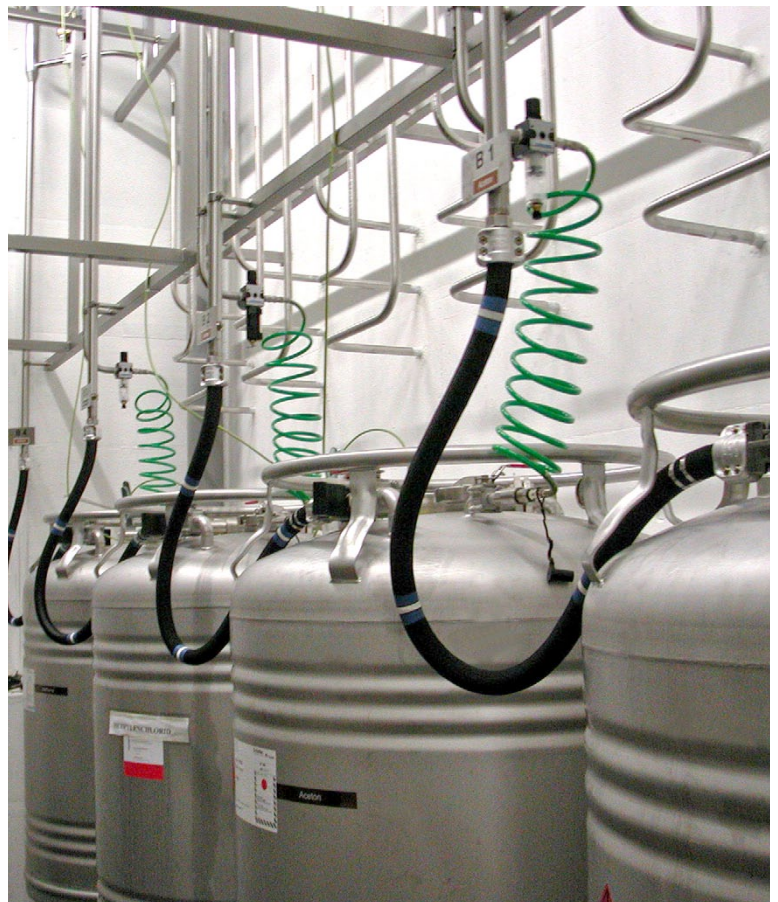
UTS universal hoses / filling of solvents with vapour recovery + solvents storage tanks - Switzerland
